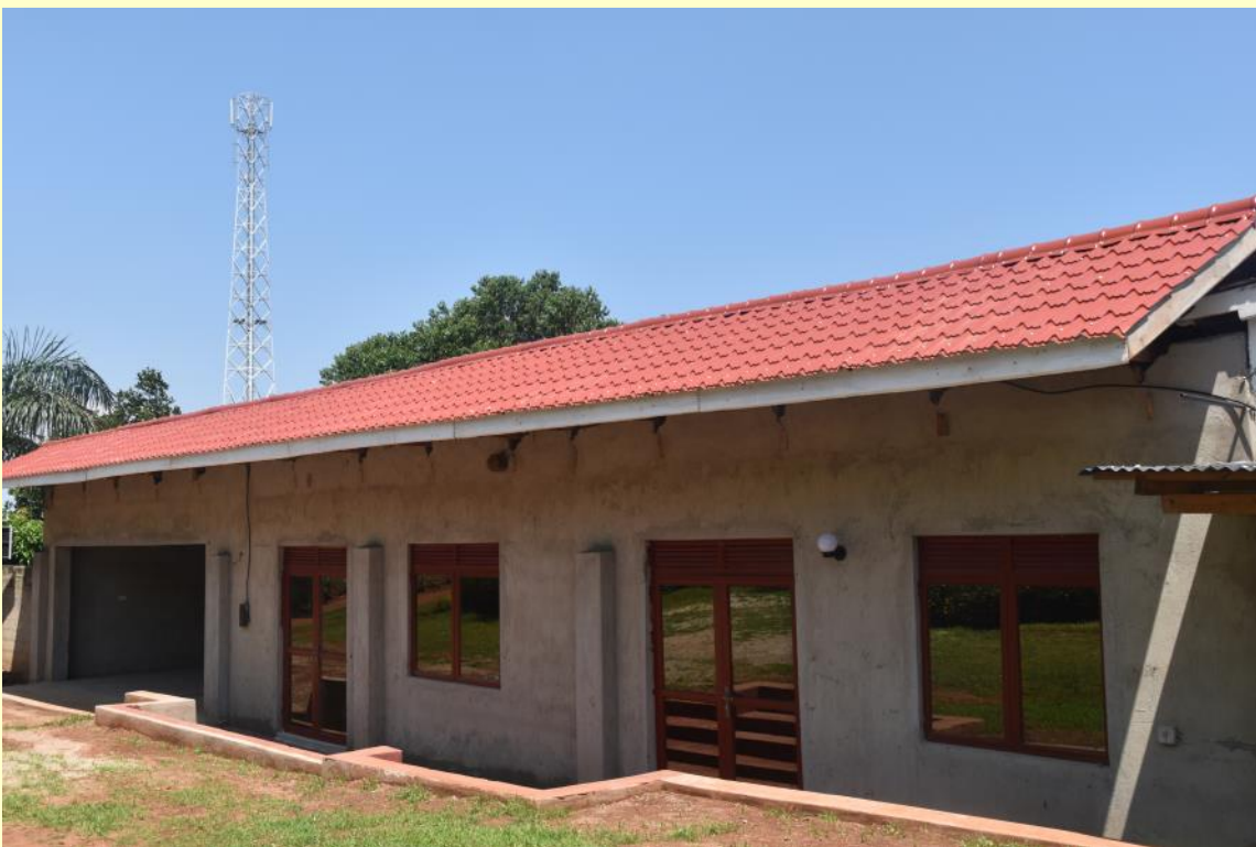
The newly constructed building with a garage., computer laboratory and dining room at its completion.
